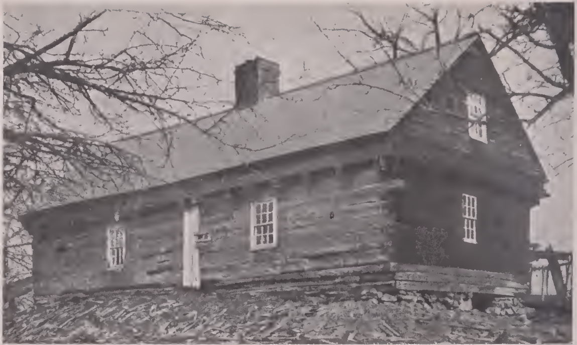
Garrison house over 252 years old, at Dover, New Hampshire. This is practically as when built. The overhang is very distinct. The chief change was made when the windows were enlarged, some 75 years ago.
